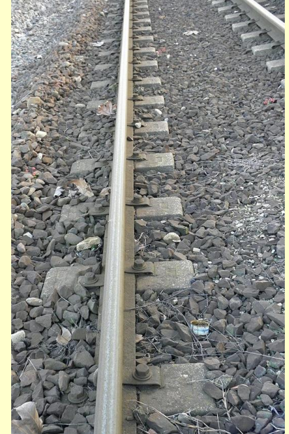
Double block reinforced concrete
