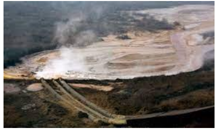
Pipes coming from a rare-earth smelting plant spew into a tailings dam on the outskirts of Baotou in China's Inner Mongolia autonomous region.
