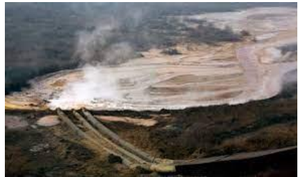
Pipes coming from a rare-earth smelting plant spew into a tailings dam on the outskirts of Baotou in China's Inner Mongolia autonomous region.
